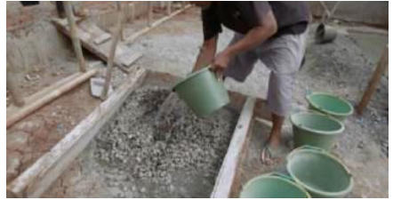
Gambar III.1 Pencampuran Beton
